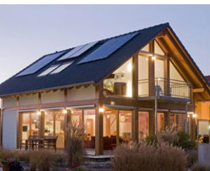
Household power station system
